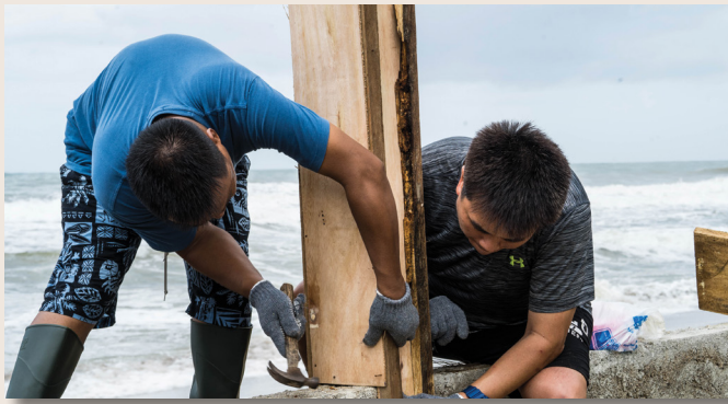
Jebsen & Jessen volunteers constructing a boardwalk.
