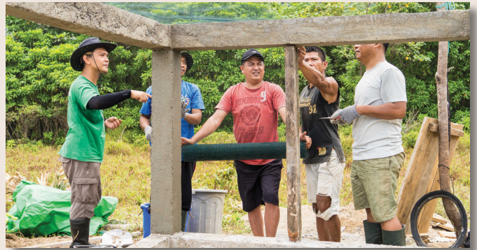
Volunteers laying the foundation for a sea turtle hatchery.
